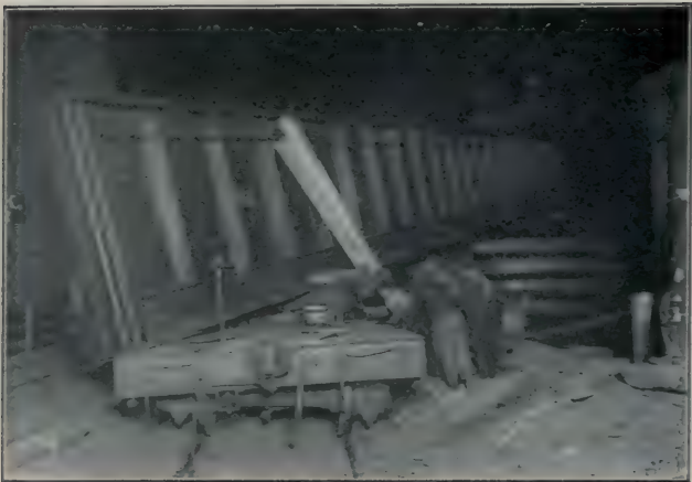
GIANT GIRDER 187 feet long. Weight nearly 120 tons
